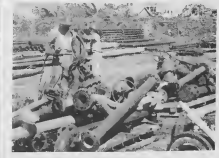
Jozef Dubero (left) and Simplicio Boekhouwer burn flanges off reclaiming pipe that has been sent to the Reclamation Yard.
